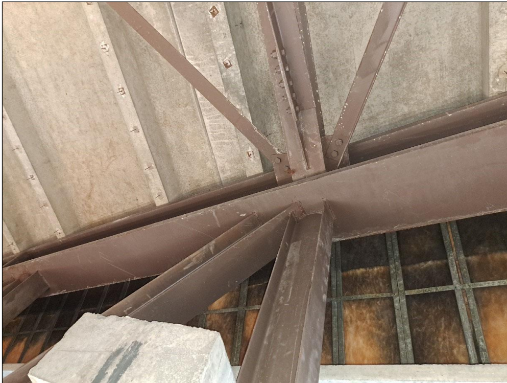
Figure 20 Centre of East side structure, "No 2 Picture".
