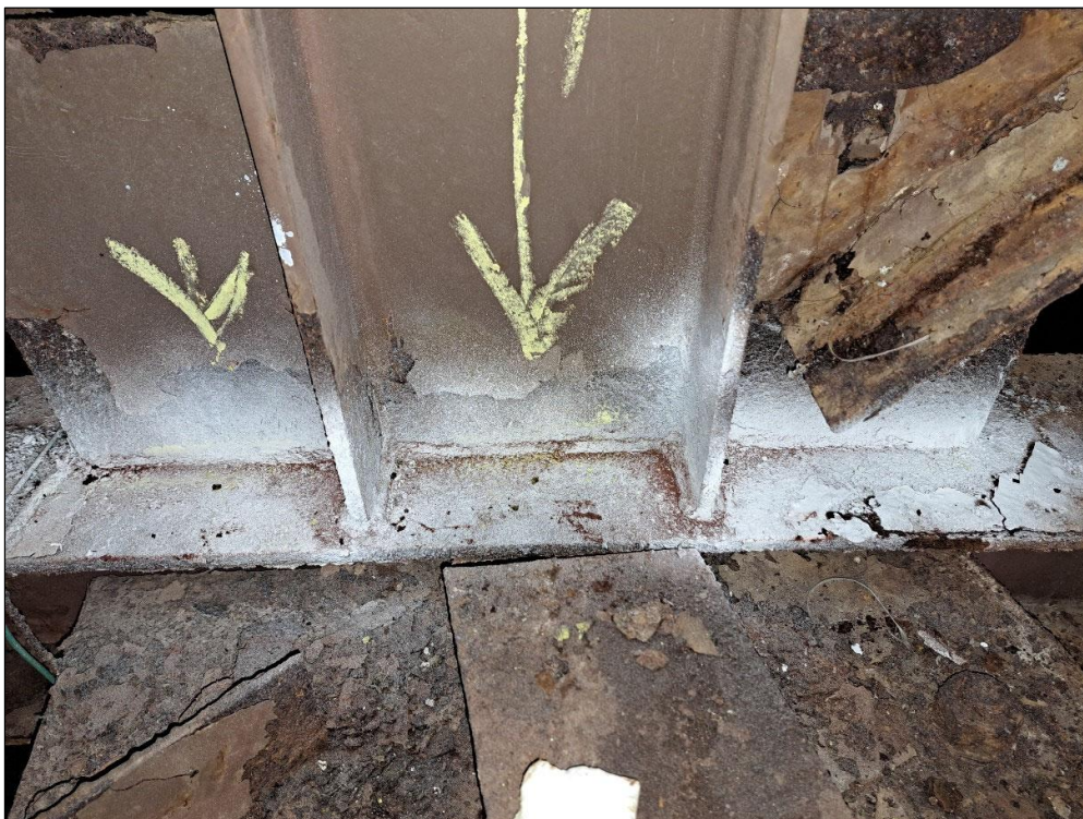
Figure 8 NW corner bottom connection. MT results.
