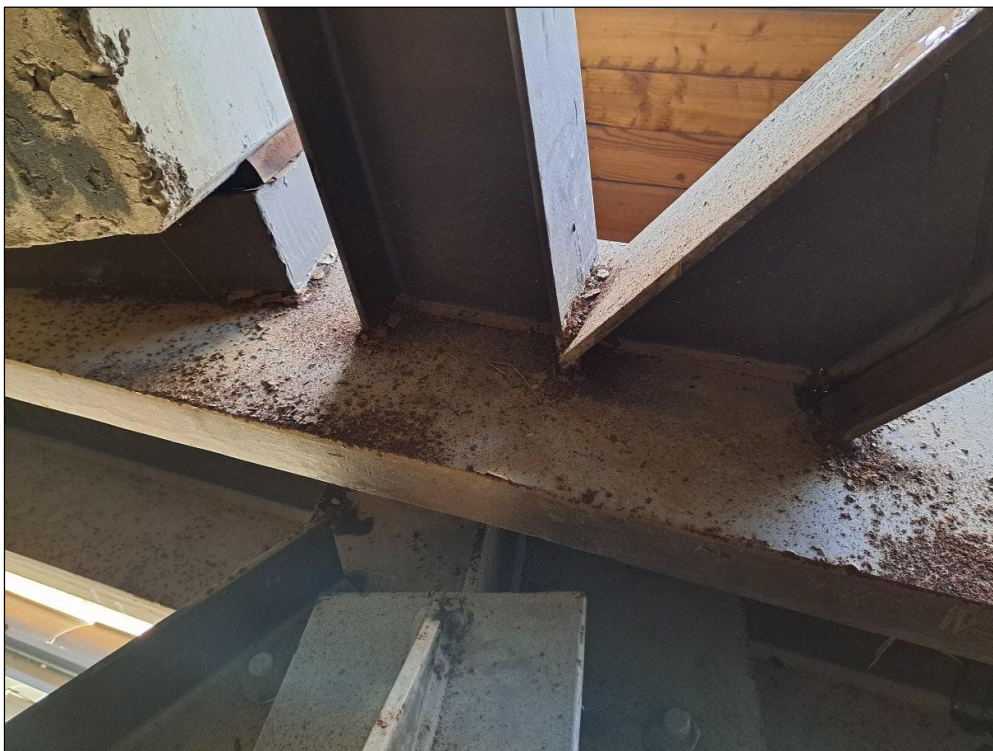
Figure 17 Centre of East side structure, "No 2 Picture".
