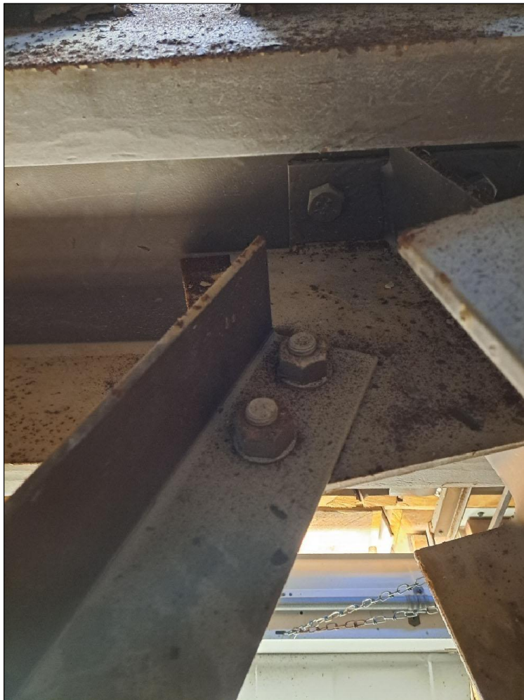
Figure 19 Centre of East side structure, "No 2 Picture".
