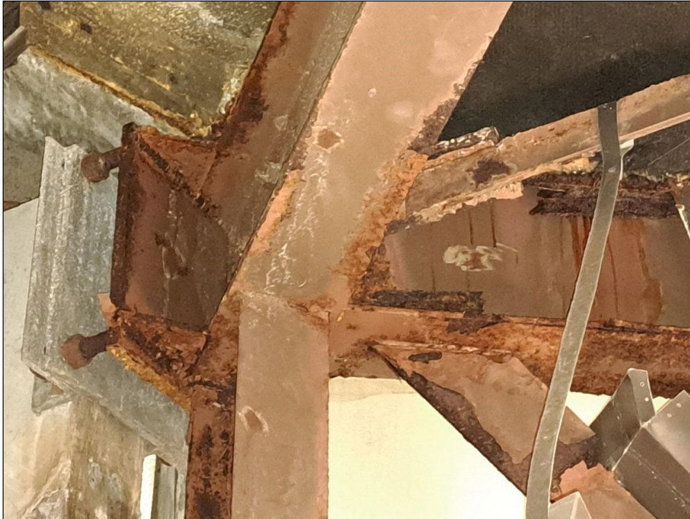
Figure 3 NW corner top connection under roof.
