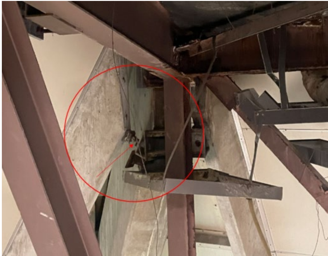
Figure 2: South West Corner Precast Panel Bolt/Pad Connection-Close-up
