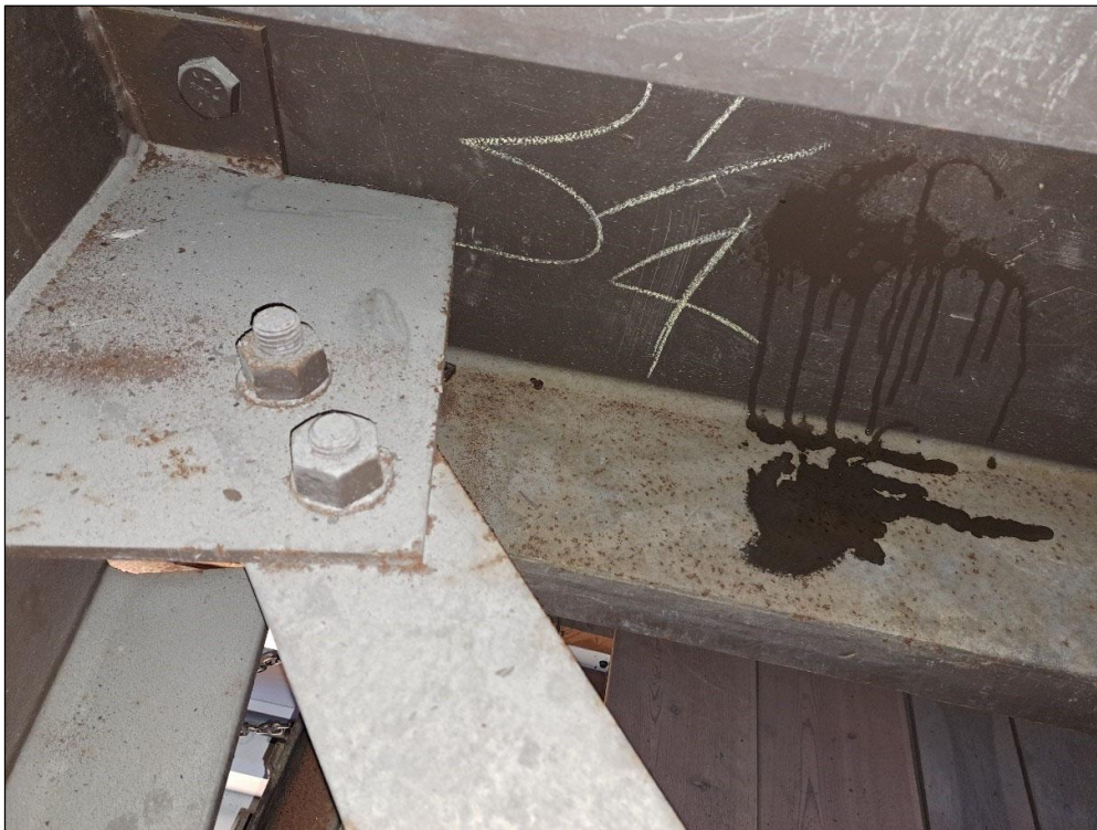
Figure 18 Centre of East side structure, "No 2 Picture".
