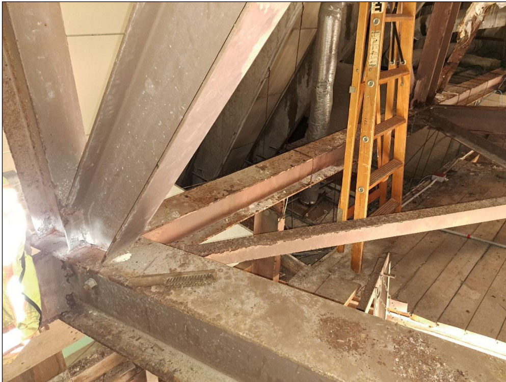
Figure 7 NW corner bottom connection. MT results.
