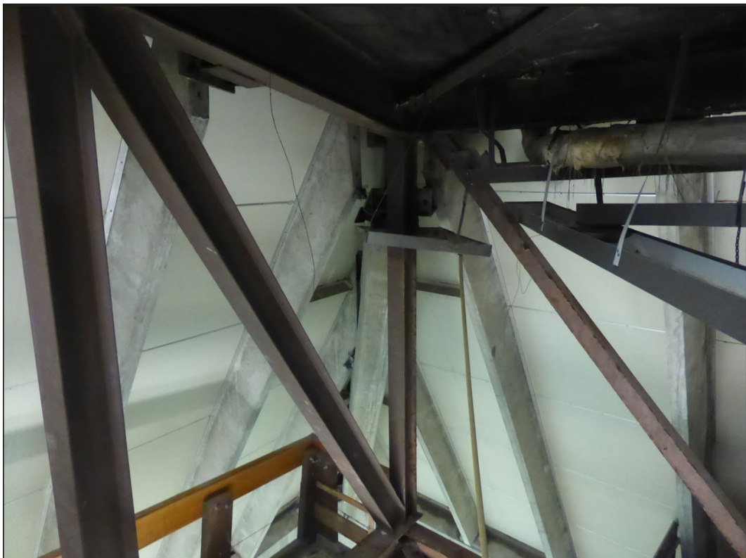
Figure 1: South West Corner Precast Panel Bolt/Pad Connection
