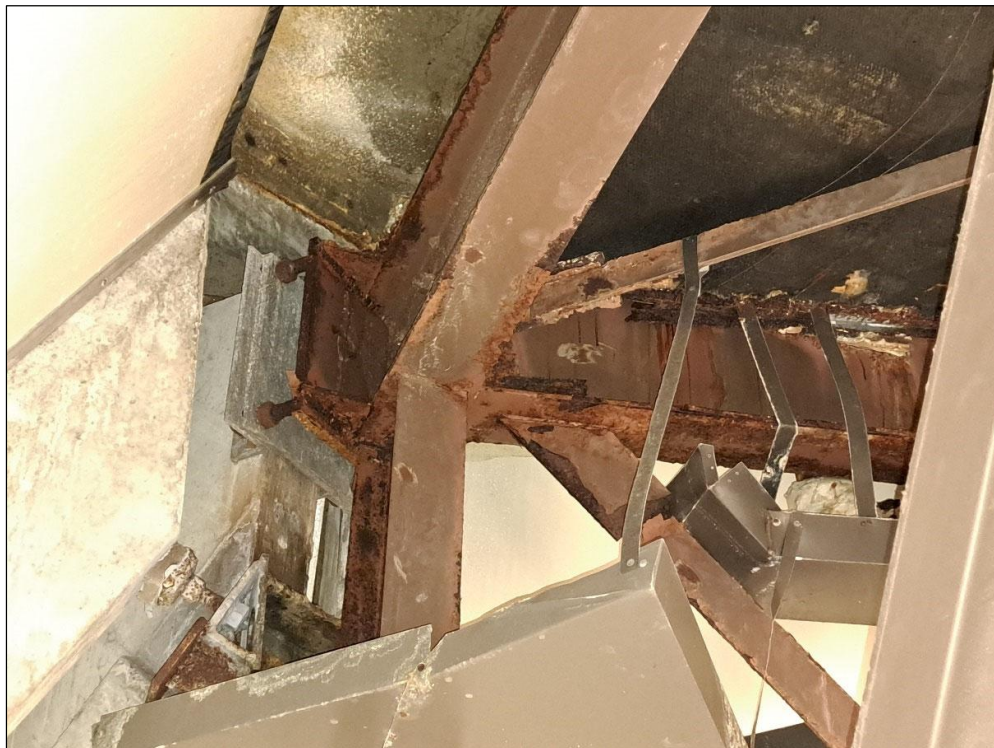
Figure 2 NW corner top connection under roof.
