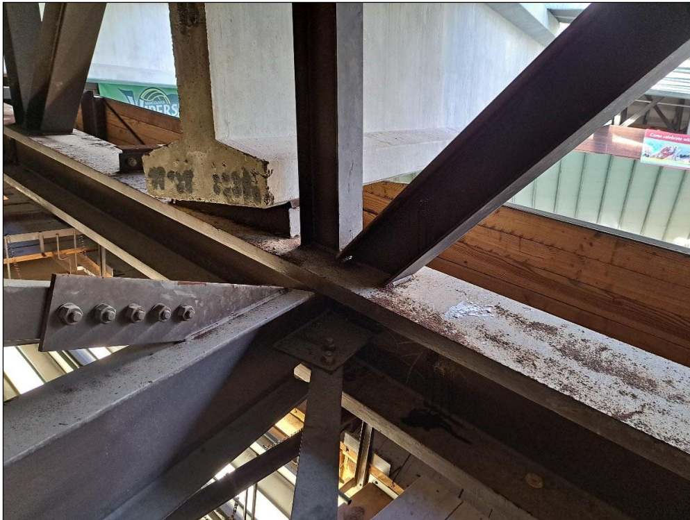
Figure 16 Centre of East side structure, "No 2 Picture".
