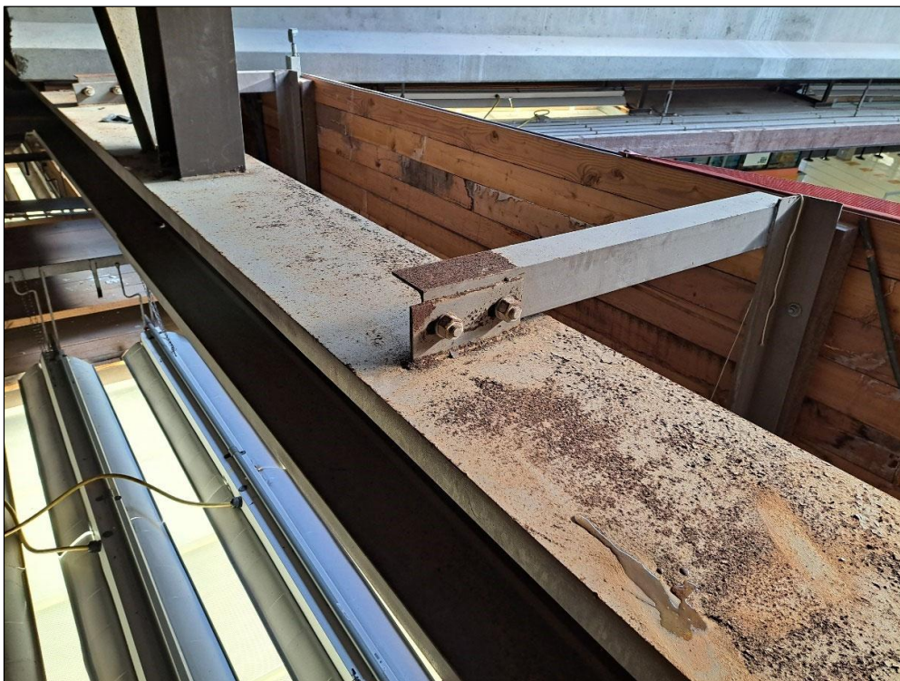
Figure 15 Centre of East side structure, "No 2 Picture".
