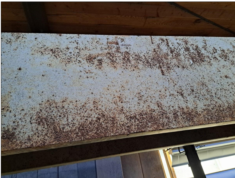
Figure 21 Centre of East side structure, "No 2 Picture".
